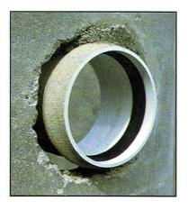
1. Core or knock out hole approximately 1+ inch larger than outside diameter of sanded manhole. Allow enough space around adapter for grout to get into.
