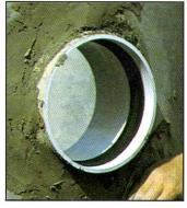
Apply a non-shrinking grout or concrete mixture in between the adapter and manhole.
